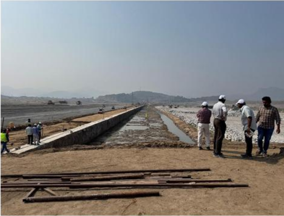
Photo 6-16: Concrete cutoff wall – GAP II Dam Cut at El. 18.5 m.
